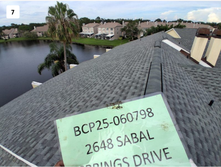
Project: 2648 Sabal Springs Dr unit 6 Date: Jul 9, 2025, 11:01 AM Creator: Lucio Roofer
