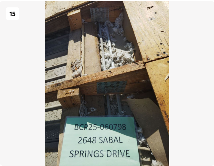
Project: 2648 Sabal Springs Dr unit 6 Date: Jul 1, 2025, 9:30 AM Creator: Lucio Roofer
