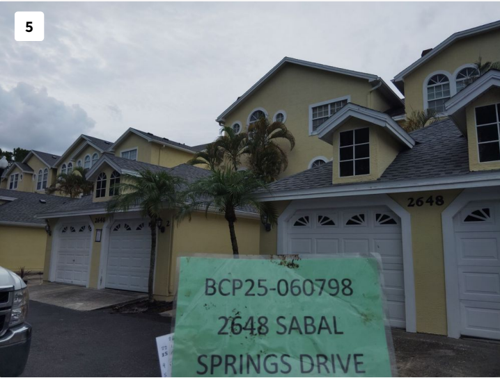
Project: 2648 Sabal Springs Dr unit 6 Date: Jul 15, 2025, 7:05 PM Creator: Lucio Roofer
