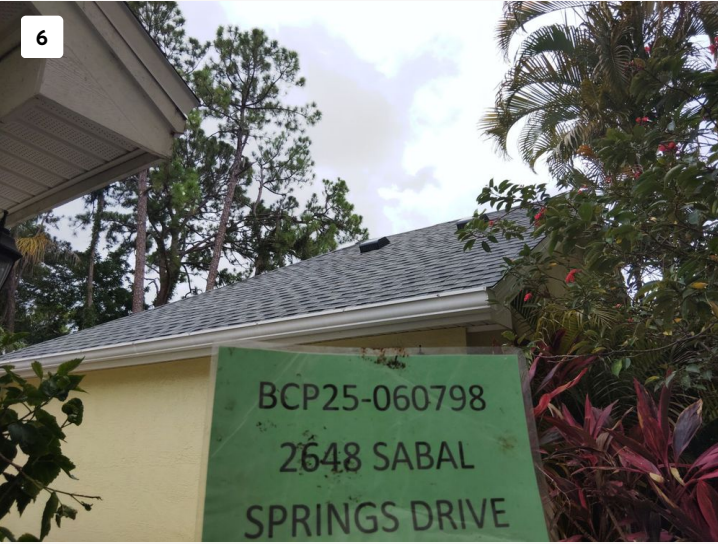
Project: 2648 Sabal Springs Dr unit 6 Date: Jul 15, 2025, 7:02 PM Creator: Lucio Roofer
