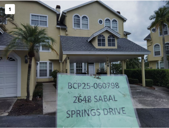
Project: 2648 Sabal Springs Dr unit 6 Date: Jul 15, 2025, 7:01 PM Creator: Lucio Roofer
