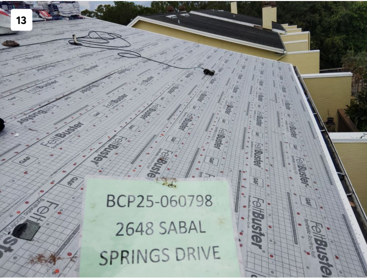
Project: 2648 Sabal Springs Dr unit 6 Date: Jul 7, 2025, 11:47 AM Creator: Lucio Roofer
