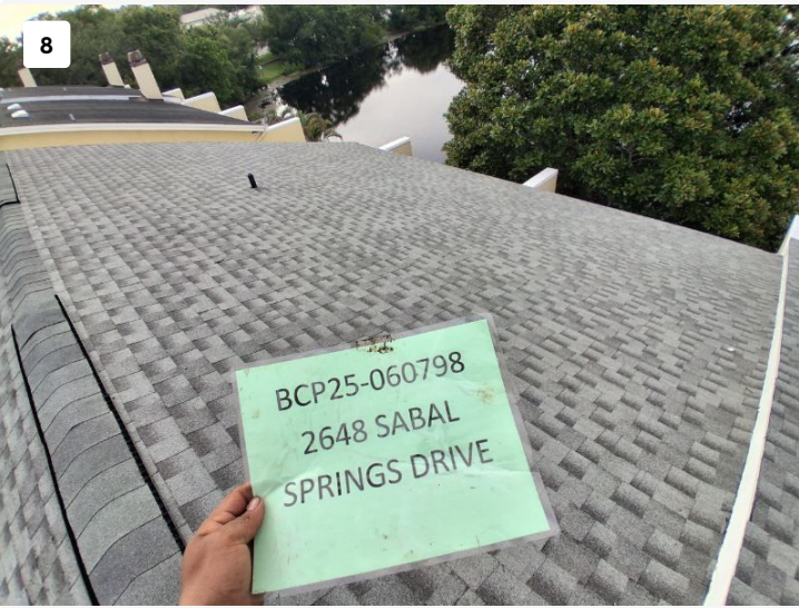
Project: 2648 Sabal Springs Dr unit 6 Date: Jul 9, 2025, 11:01 AM Creator: Lucio Roofer
