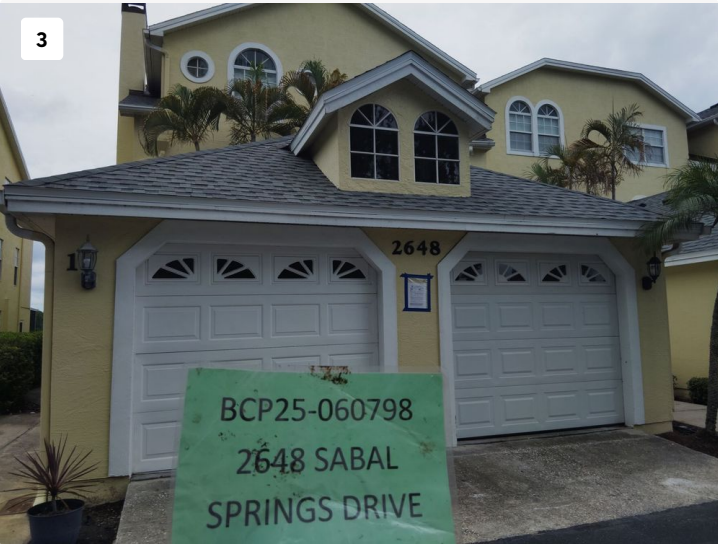
Project: 2648 Sabal Springs Dr unit 6 Date: Jul 15, 2025, 7:04 PM Creator: Lucio Roofer
