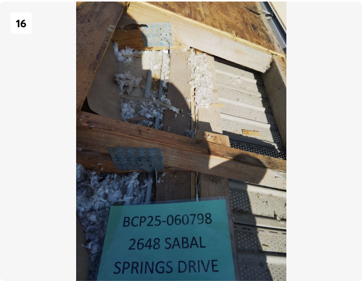
Project: 2648 Sabal Springs Dr unit 6 Date: Jul 1, 2025, 9:29 AM Creator: Lucio Roofer
